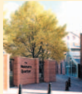
Hull Museums Quarter Orientation Centre - Kingston upon Hull - a successful controlled response with a challenging refurbishment and extension brief.
