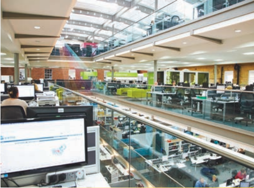
The new four storey office structure
