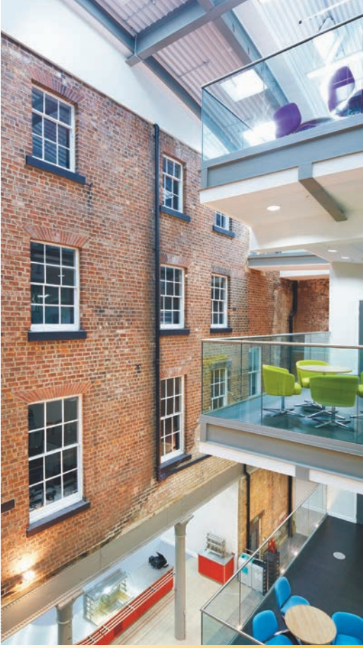
A light well between the old façade and the new offices
