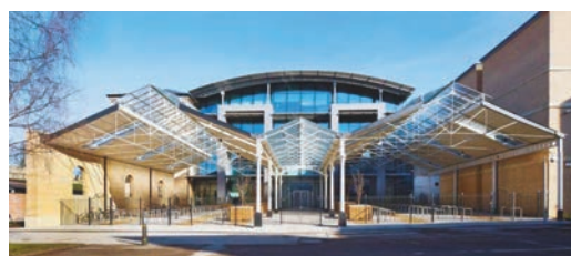
The approach to the building reflecting the railway heritage
