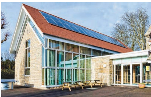
New school hall with corner glazing and glazed link and Purbeck stone finish
