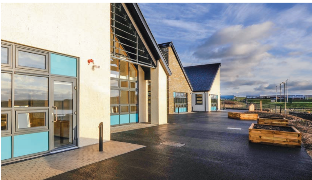
The limited palette of materials providing a contemporary solution
