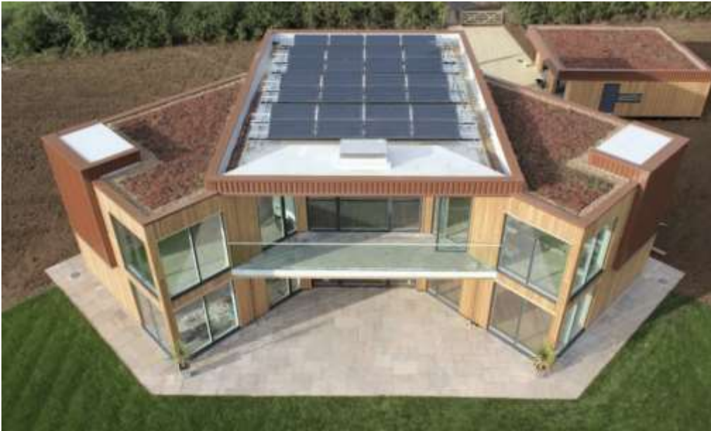
Rooftop with PV-thermal (PVT) panels collecting heat and generating electricity
