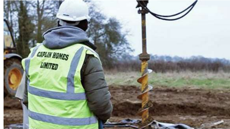
Drilling shallow 1.75m boreholes
