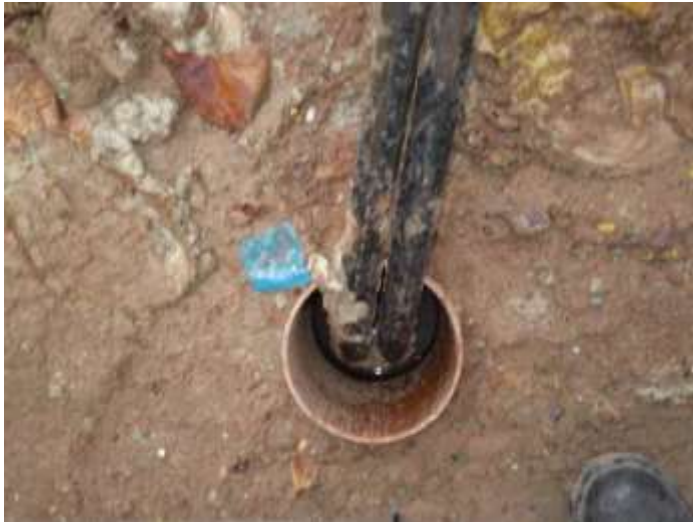
Drilling at DMU for Hugh Aston Building (this building)
