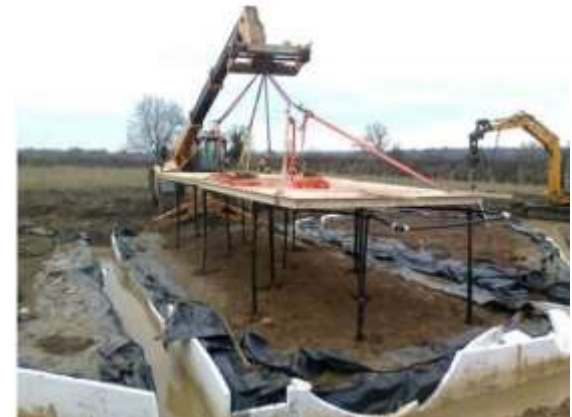
Dropping pipe network into holes to store solar heat
