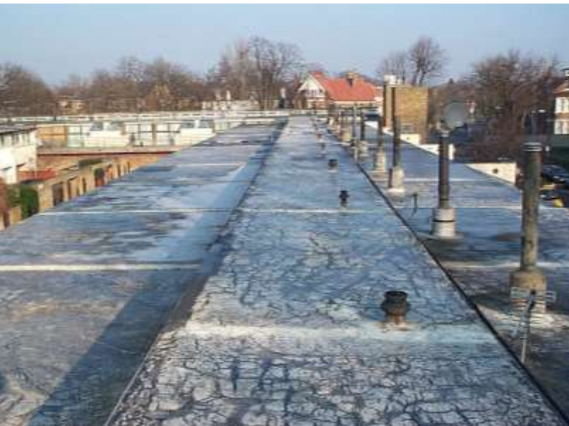
Existing roof conditions
