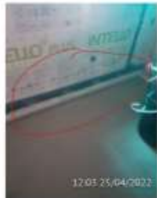
Snag 3 - FN 01 Study Assigned To LTF Incorrect detail, intello plus membrane should finish flush with screed and the Contega taped from screed to intello membrane
