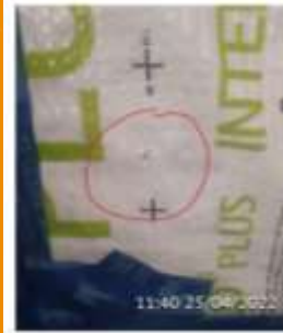
Snag 3 - FN 01 Study Assigned To LTF Incorrect detail, intello plus membrane should finish flush with screed and the Contega taped from screed to intello membrane
