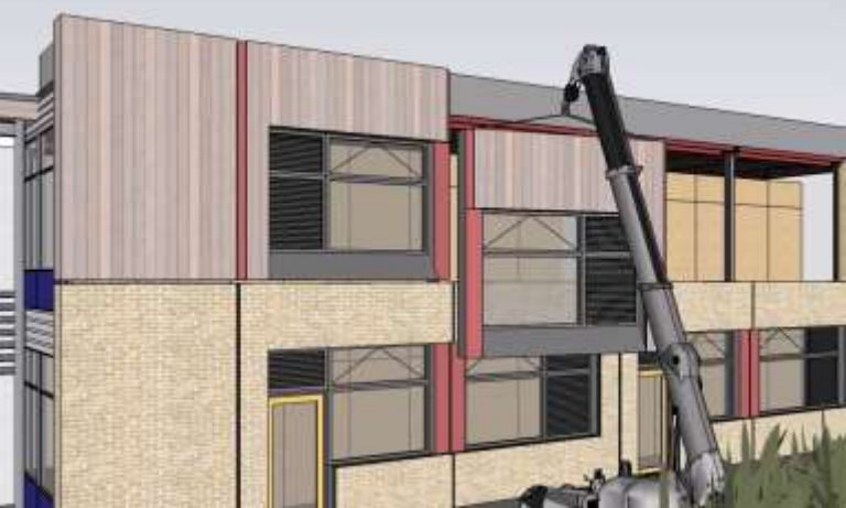
Installation of GF Panels with Spider Crane
